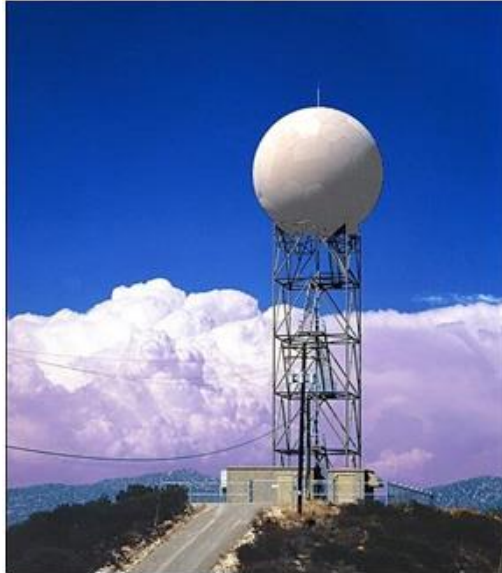
Figure 2: Image of NEXRAD radar site with antenna tower and radome. Image Source: ( https://www.ll.mit.edu/mission/aviation/faawxsystems/nexrad.html )
