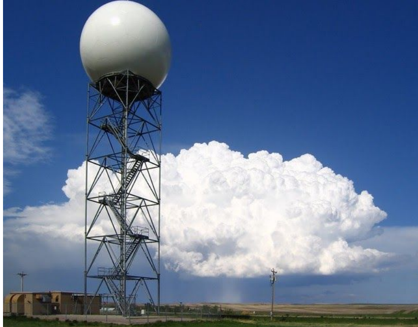
Figure 3: Image of NEXRAD radar site with an antenna tower and radome. (Image source: NOAA Photo Library )
