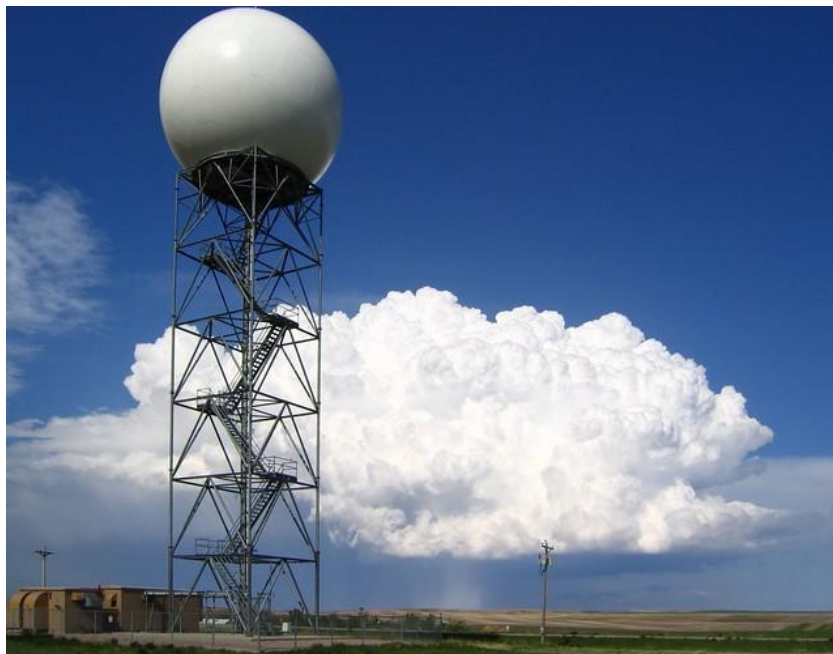
Figure 3: Image of NEXRAD radar site with an antenna tower and radome. (Image source: NOAA Photo Library )
