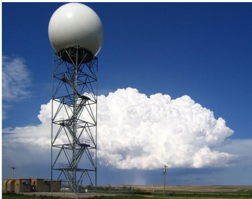
Figure 3: Image of NEXRAD radar site with an antenna tower and radome.
